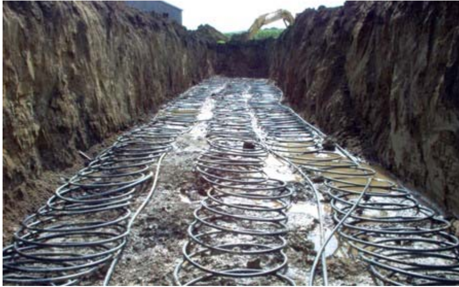
Figure 2-3 Slinky Ground Loop Heat Exchanger for a Small 3-ton Heat Pump System (Source: Wikipedia; Mark Johnson photo)
