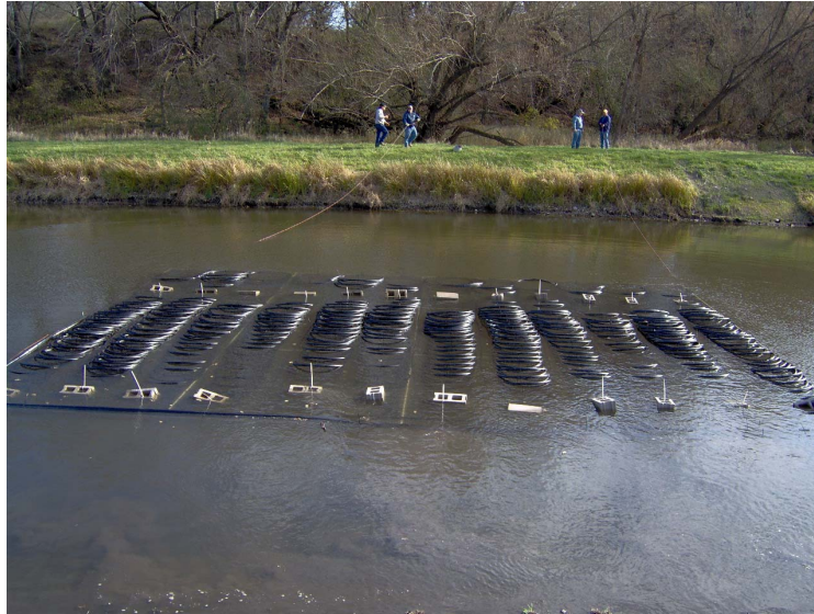
Figure 2-6 Picture of a 12-ton Pond Loop Heat Exchanger Before it is Sunk to the Bottom of the Pond
