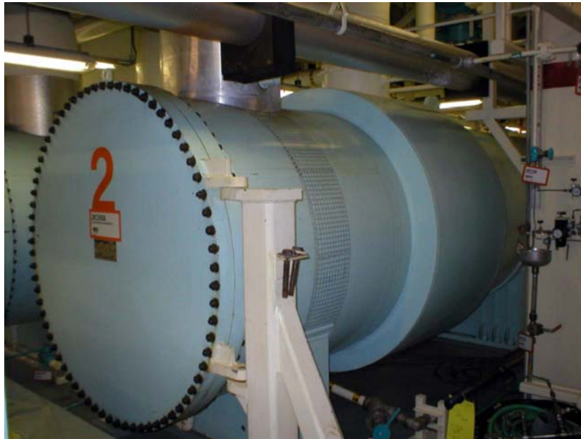
Figure 1-1 Component cooling water system heat exchanger
