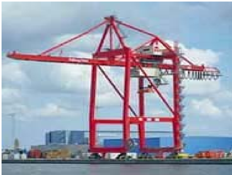
Figure 3-5 A KoneCranes Ship to Shore Crane
