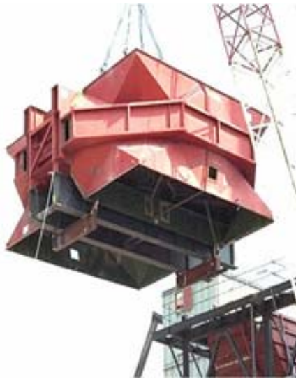
Figure 1-1 Typical Regenerative APH (courtesy: Howden)
