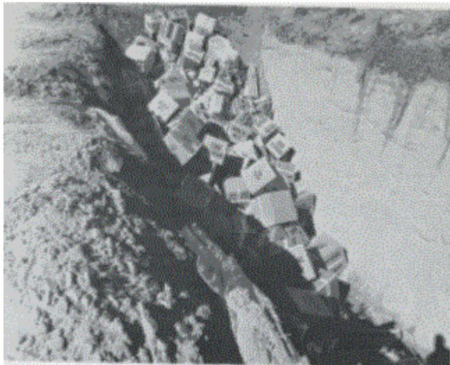
Figure 4-1 Random Placement (Kick-and-Roll) Disposal of Un-stabilized Waste (circa 1970)
