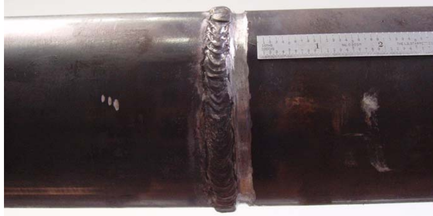
Figure 3-2 Flaw #1, 360° Groove Adjacent to Girth Weld
