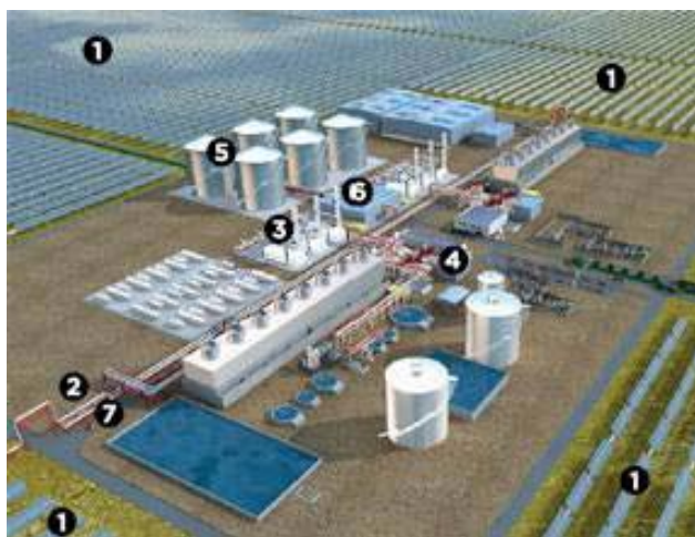
Figure 2-9 Artist's Rendering of APS Solana Power Plant; Molten Salt Storage Tanks are Labeled “5” 6
