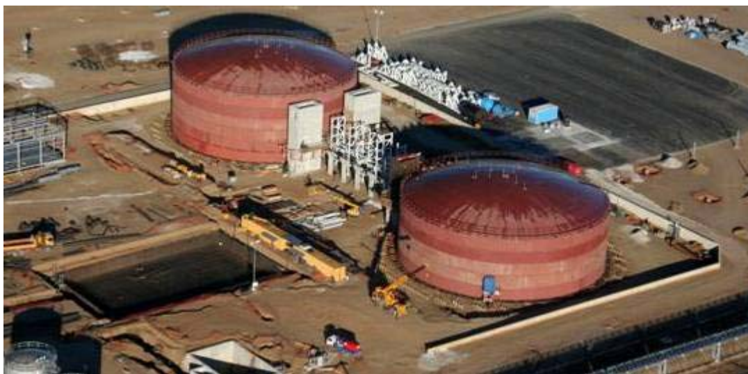
Figure 2-8 Thermal Storage Tanks under Construction at Andasol 1 (2007)
