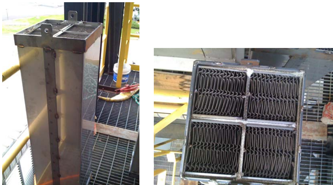
Figure 4-2 Photograph of Pilot Catalyst Module (side and top views)
