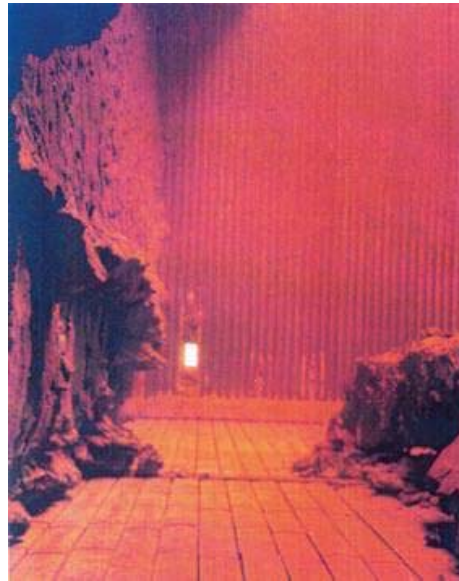
Figure 5-2. Boiler Slagging After Operating for 4 Days on Urban Tree Trimmings (Source: T.R. Miles).
