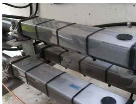
Figure 5-2 Flexible magnetic coupler with additional protection installed on cable outside jackets
