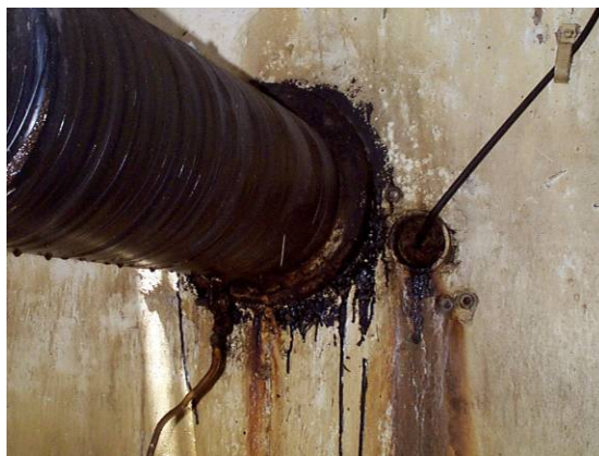
Figure 3-3 Distributed Temperature-Sensing Optical Fibers in a 3-Inch PVC Conduit Adjacent to a Pipe-Type Cable Pipe
