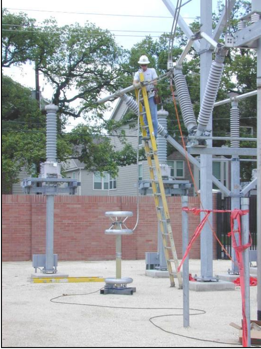
Figure A-5 Standard Capacitor Connection in Midtown Substation
