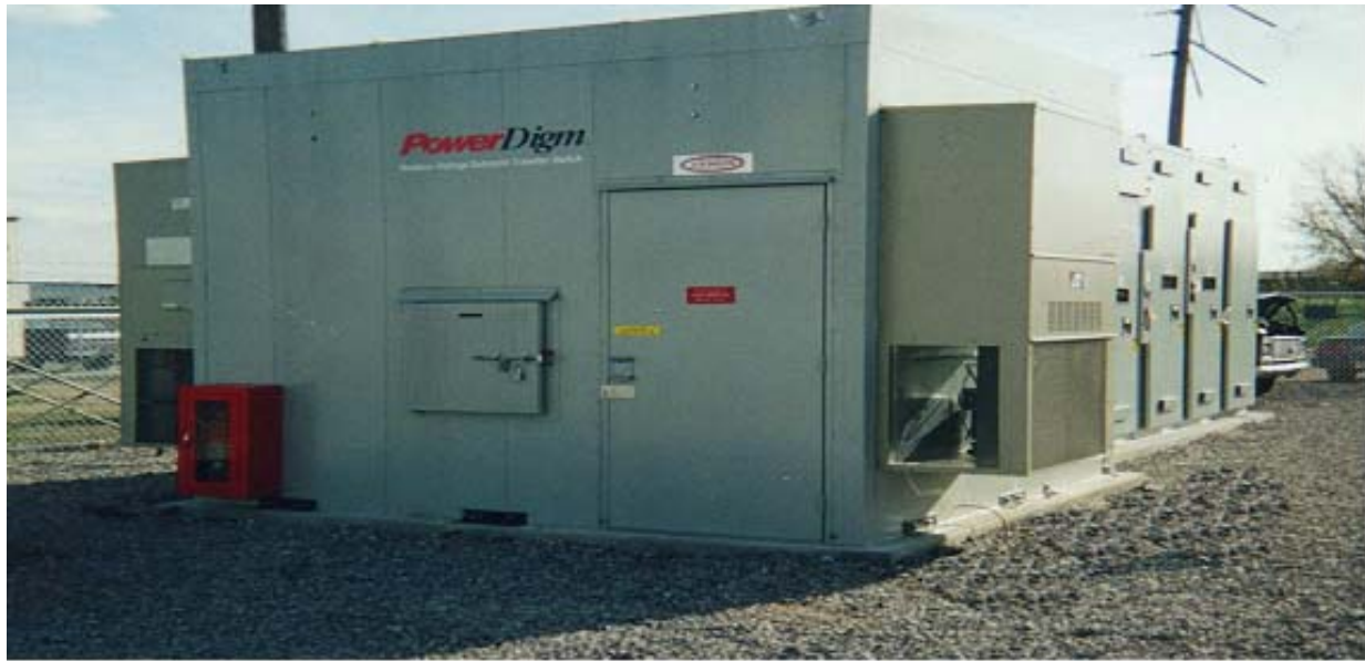
Figure 3-3 15kV, 600A Outdoor Installation for Ford Motor, Detroit Michigan
