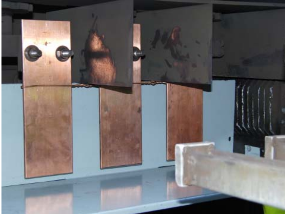
Figure 1-5 Configuration with a Conducting Plate Behind and Below the Bus Bars
