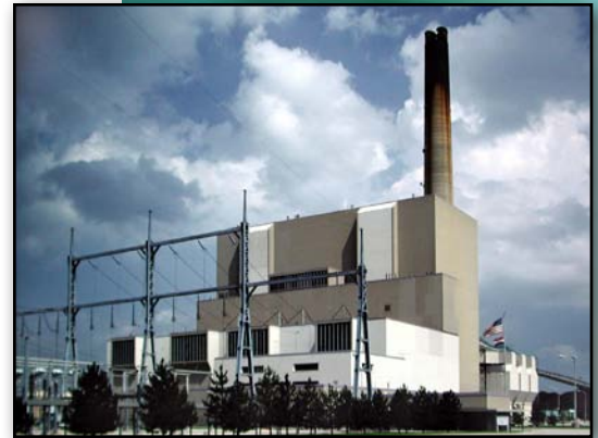
Rush Island Power Plant
