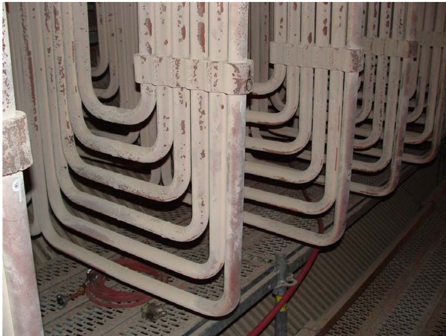
Figure 1-1 Pendant of secondary superheat outlet tubes
