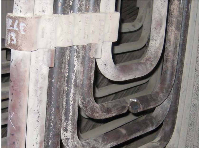
Figure 1-10 shows a tube cut for removal of magnetite
