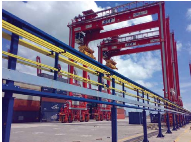
Photo 2. Conductix-Wampfler Conductor Rail System
