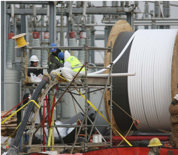
Figure 1: Installation of a superconducting DC cable (manufactured by Southwire) at an American Electric Power substation. Photo courtesy: Southwire
