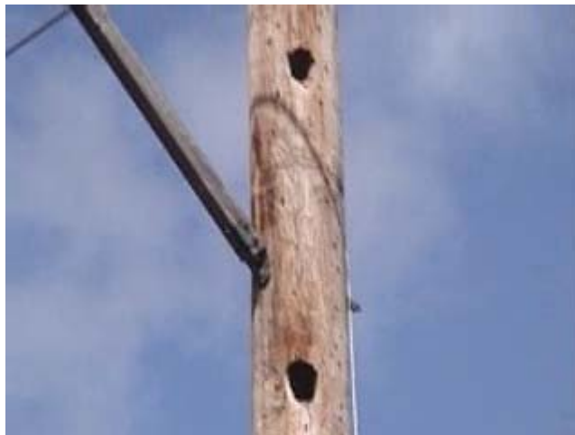
Figure 1-2 Pileated Woodpecker Roosting Cavities in a H-Structure Transmission Pole on New York State Electric and Gas (NYSEG) Hammondsport Line 04 May 2005
