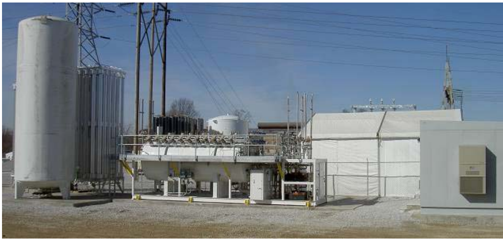
Figure 2-5 Open cycle cooling system showing storage tank, vaporizer, cold box and control building Used with permission from Southwire Company
