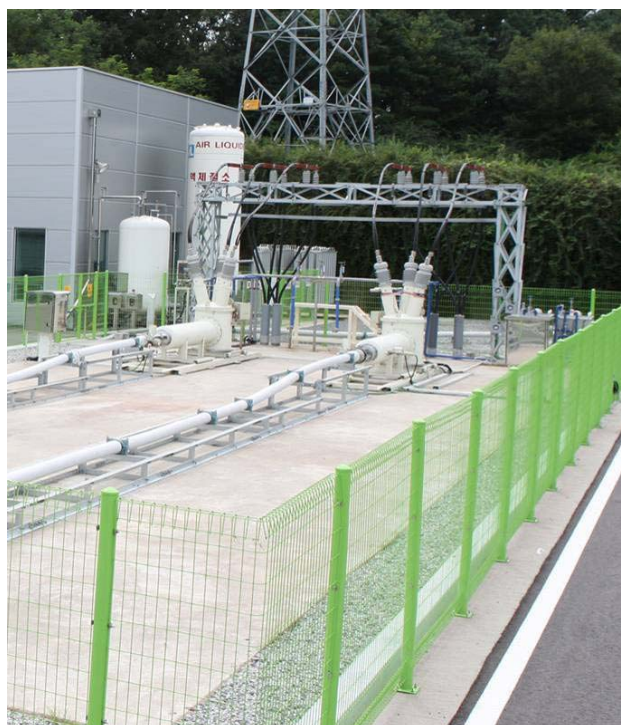
Figure 3-4 Conceptual drawing of the 22.9kV HTS cable terminations in I'cheon City, Korea Source: KEPRI-EPRI Joint Superconductivity Conference, November 16–18, 2009, Daejeon, South Korea
