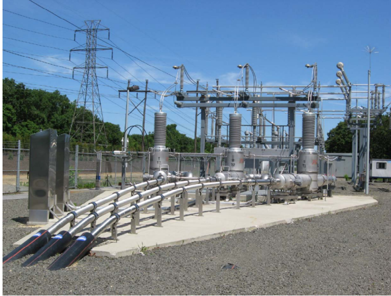
Figure 2-1 North terminations of the 138 kV, 600 m HTS transmission cable at Keyspan/LIPA Source: Demonstration of a Pre-Commercial Long-Length HTS Cable System Operating in the Power Transmission Network, 2009 DOE Peer Review, August 4, 2009. Alexandria, VA
