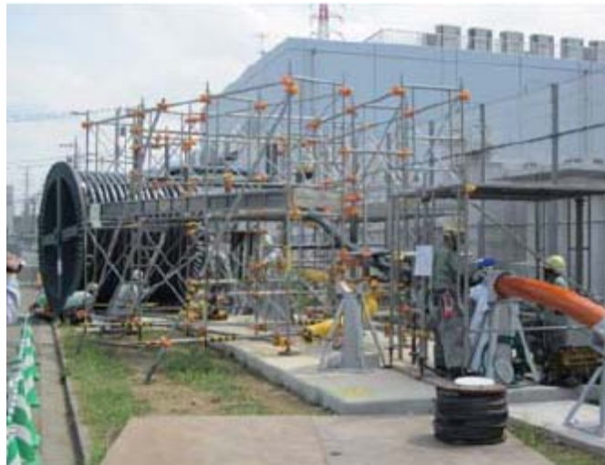
Figure 2-10 Installation of 66 kV (200 MVA) HTS cable system in Yokohama, Japan Used with permission from TEPCO
