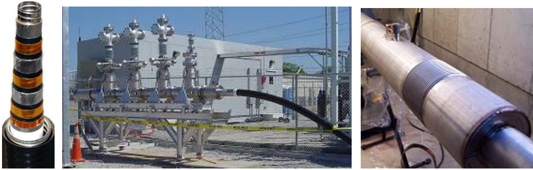
Figure 2-4 HTS Triax ® cable (left), termination (center) and splice (right) Used with permission from Southwire Company
