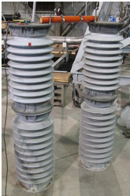
Figure B-8 2 Stacks of 2 Insulators Each, with a Test Piece Mounted on Top.
