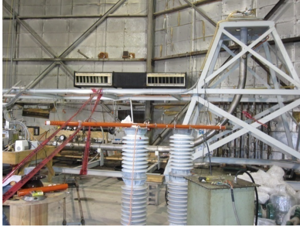
Figure 5-14 View of the Test Setup for Flashover Tests.
