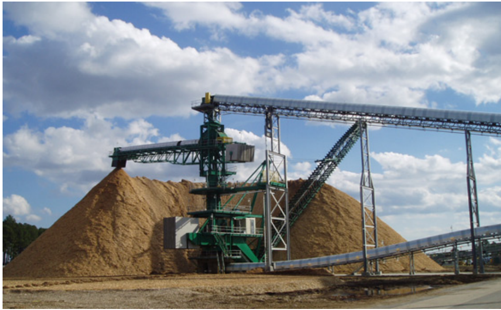
Figure 4-5 Biomass Storage and Reclaim System
