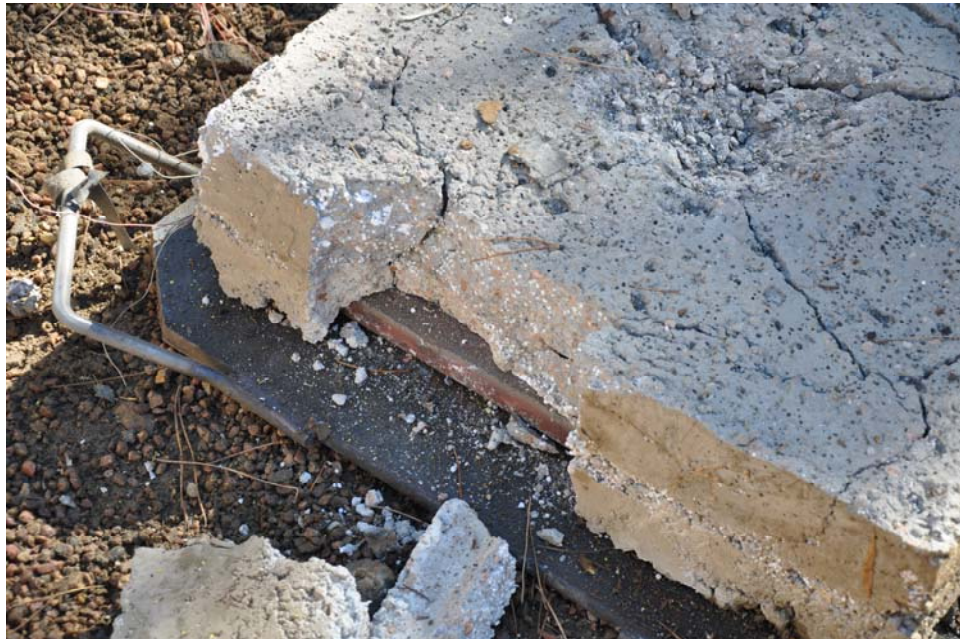
Figure 3-4 Photograph of damaged light concrete experimental setup after blasting.
