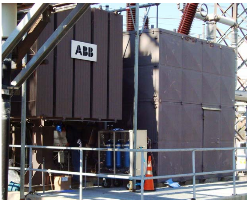
Figure 4-1 On-line Corrosive Sulfur Removal Prototype Unit Installed on a Shunt Reactor.
