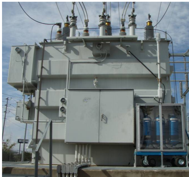
Figure 3-1 On-line Corrosive Sulfur Removal Prototype Unit Installed on a 30MVA Transformer.
