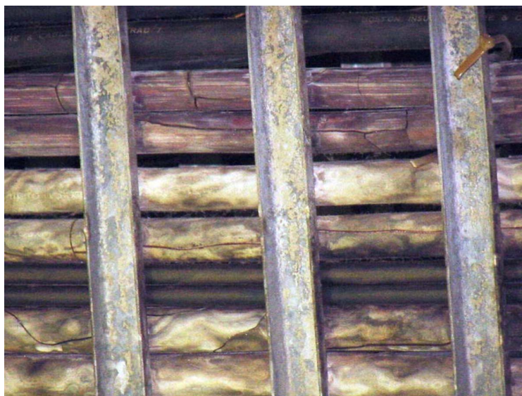
Figure 2-9 Neoprene and CSPE Jacketed Cables in the Same Tray
