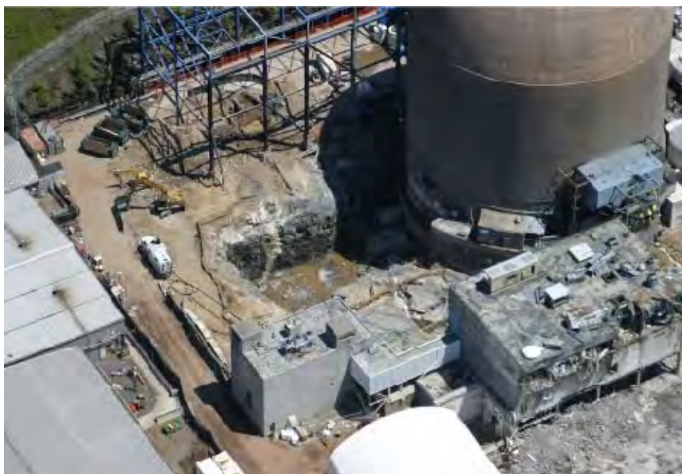
Figure 4-1 PAB Excavation at CY
