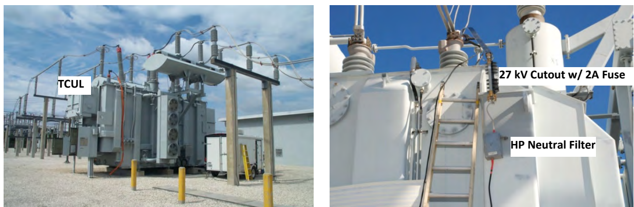
Figure 11-6 First OLFRA Installation on a Three-Phase Auto-Transformer with All Three Phases in One Tank
