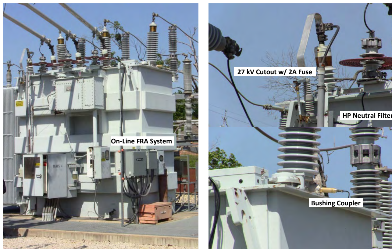
Figure 11-27 OLFRA Installation on a Delta-Wye Transformer with an LTC
