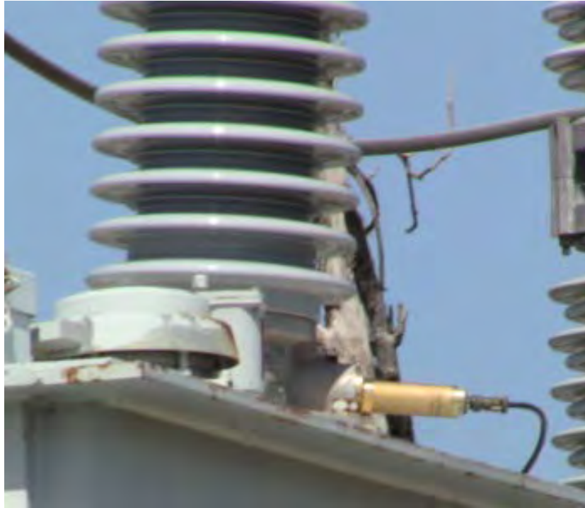
Figure 6–2 Bushing Tap Coupler in a Bushing Capacitance Test Tap
