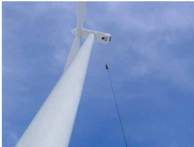
Figure 4-3 Oil change hose hoisting Courtesy of Sage Oil Vac
