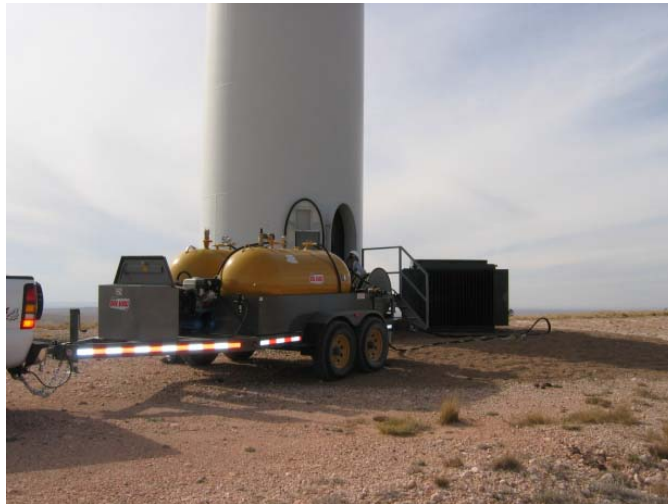
Figure 4-2 Mobile unit at tower base Courtesy of Sage Oil Vac
