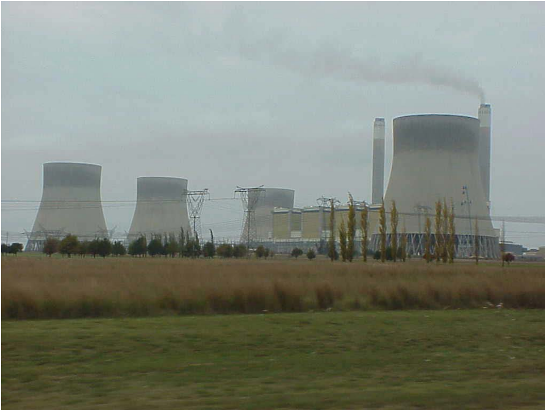
Figure 2-11 Indirect dry cooling system with natural draft towers; Kendal Station, South Africa
