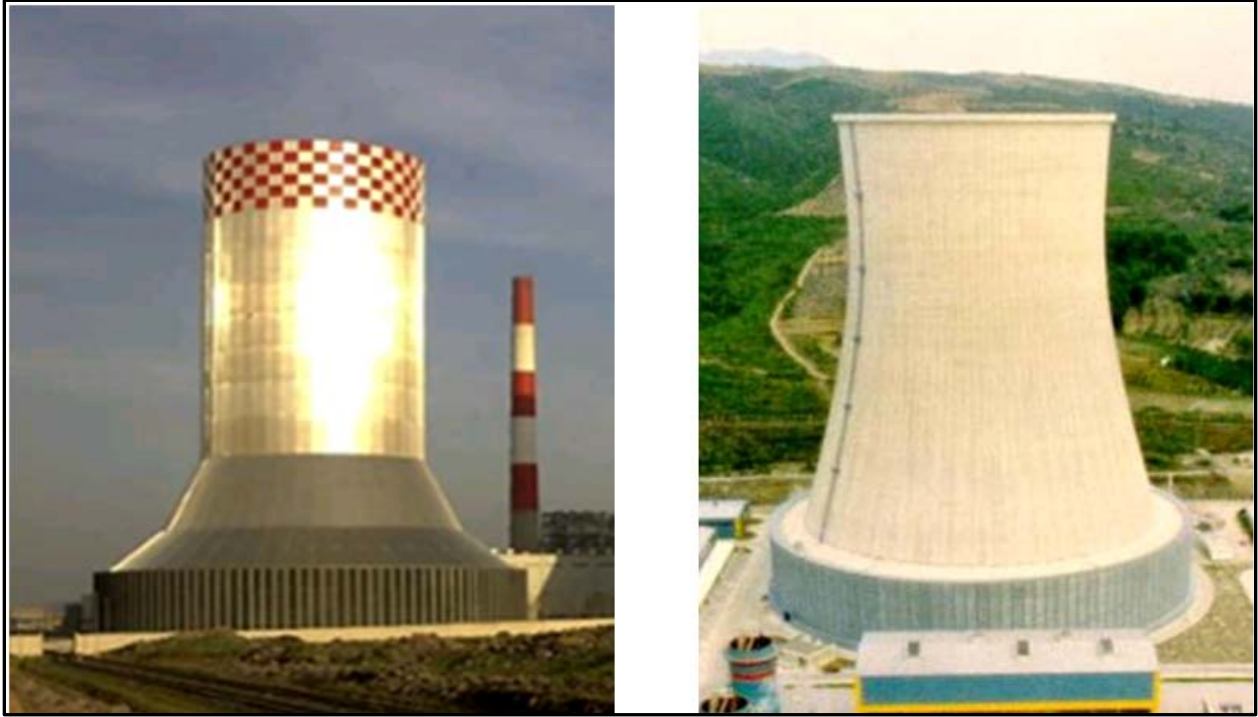
Figure 2-10 Natural-draft towers with peripheral ACHEs
