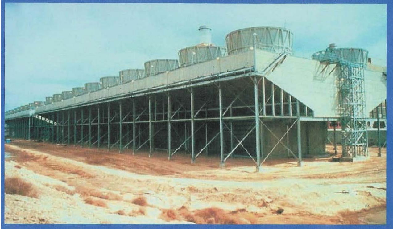
Figure 2-24 Photograph of integrated water conservation tower (Public Service New Mexico San Juan Generating Station Unit 3)
