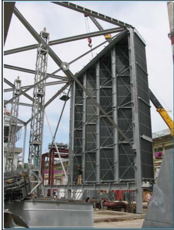
Figure 2-7 Cooling deltas being positioned on side of ACHE
