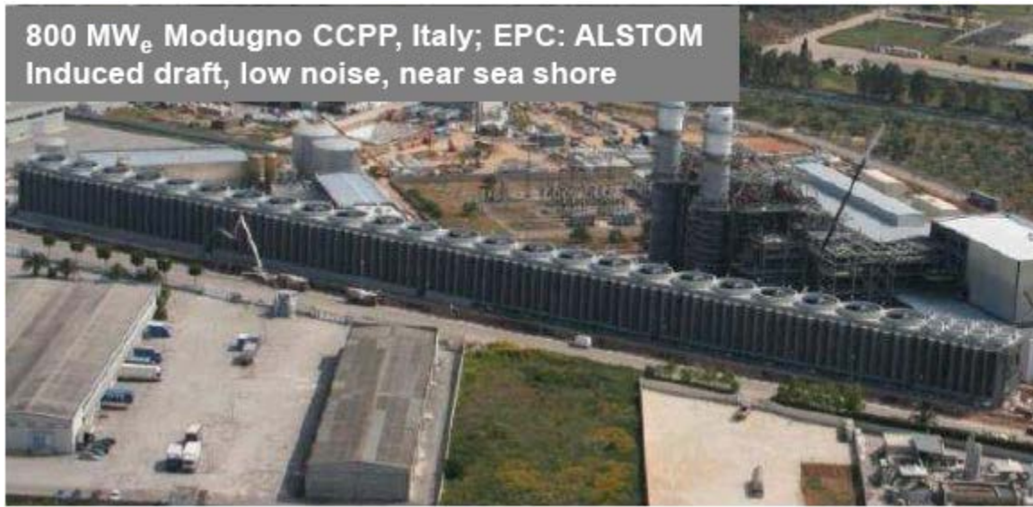
Figure 2-17 System with mechanical-draft dry cooling tower
