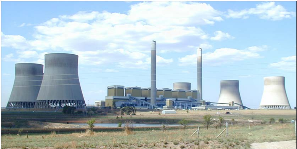
Figure 5-4 Kendal Power Station
