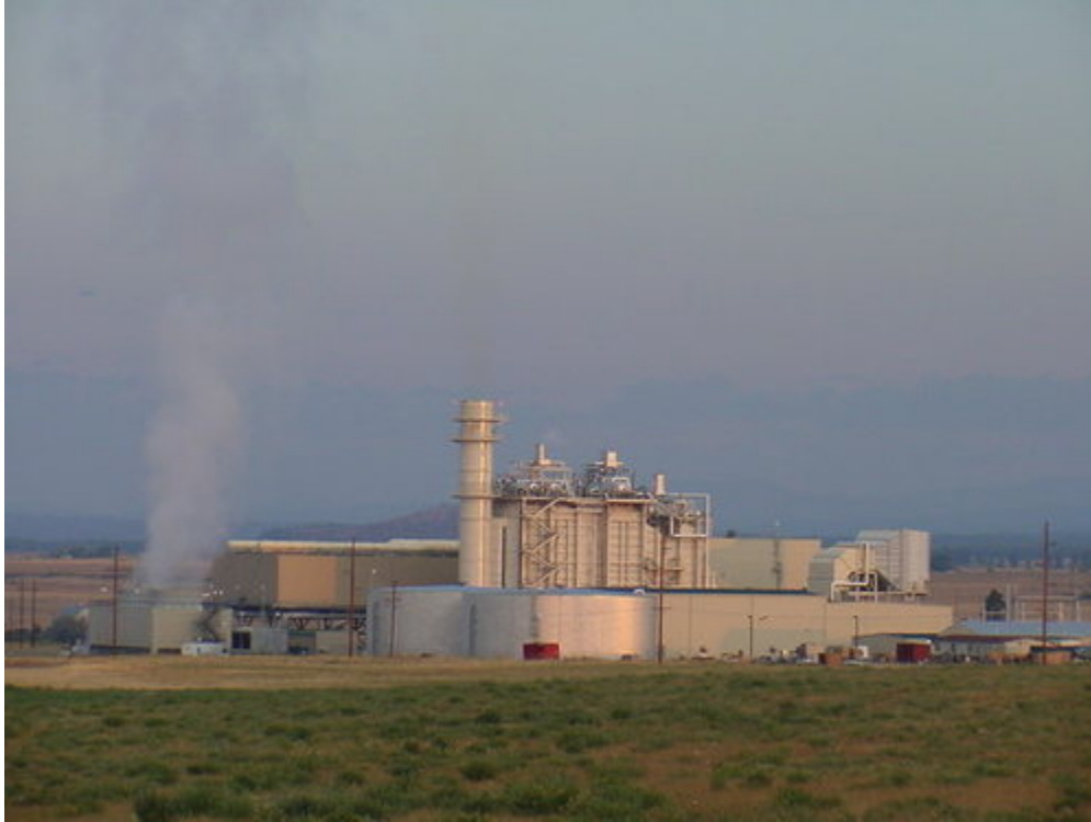
Figure 2-21 Hybrid water-conservation cooling system (shown with a 10 cell air-cooled condenser and a 2 cell wet cooling tower) (from http://www.panoramio.com/photo/2293438 )
