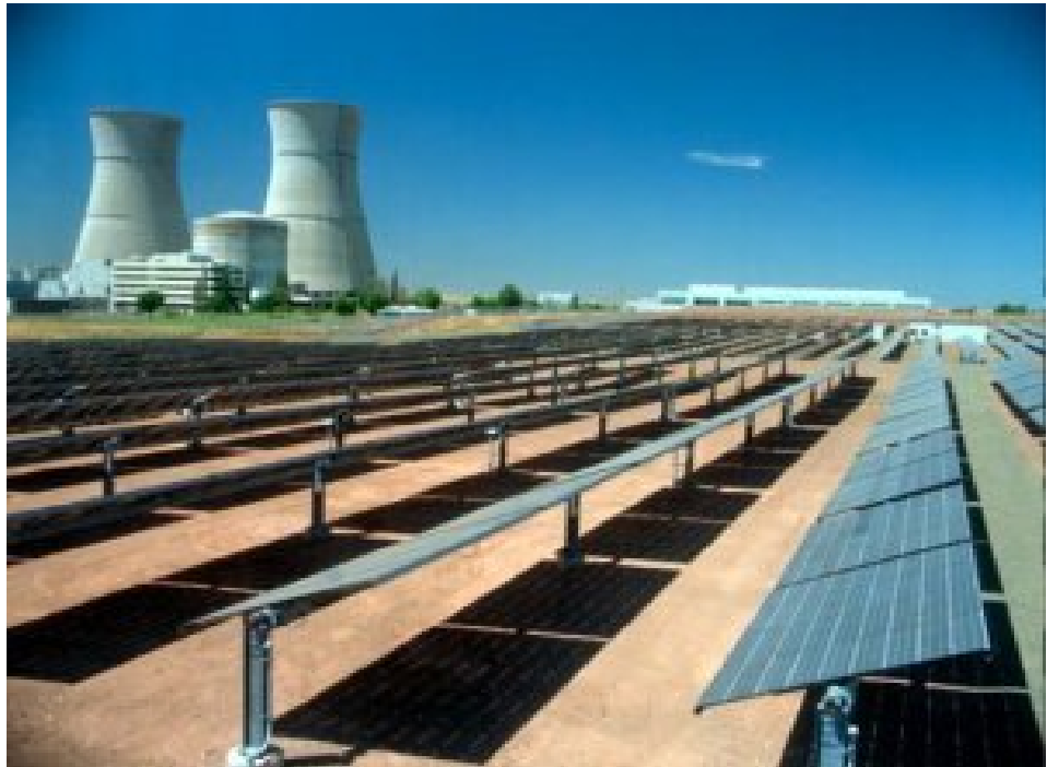
Figure 3-3 Rancho Seco Photovoltaic Generating Facility
