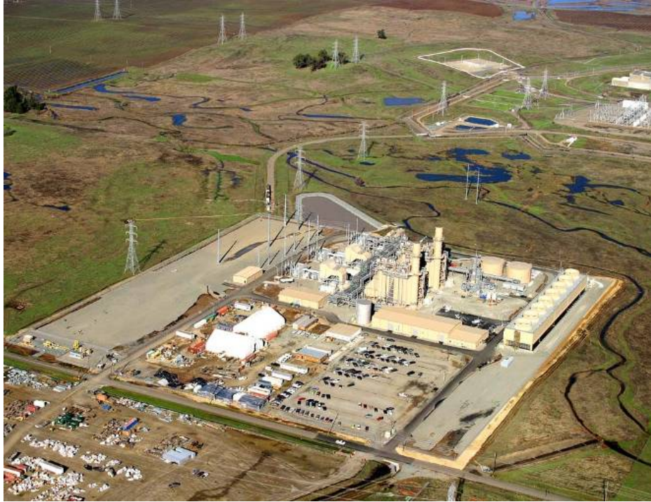
Figure 3-4 Rancho Seco Combine Cycle Power Plant
