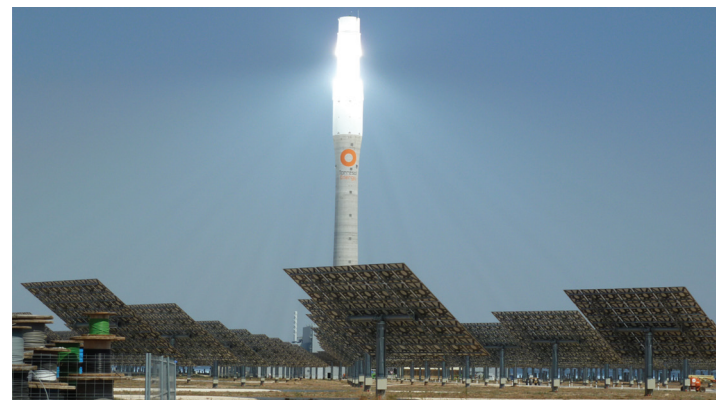
Figure 7: Heliostats focus sunlight on the receiver (Source: T. Peterson)
