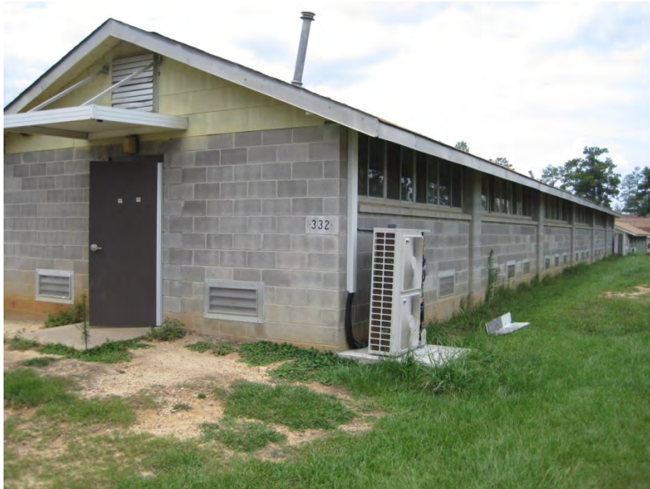
Figure 5-8 Enlisted Barracks Treatment (DHP) Building
