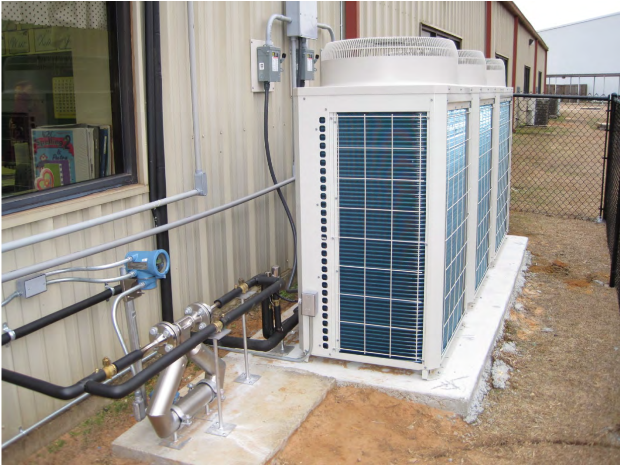
Figure 4-21 VRF System Installed at Site B
