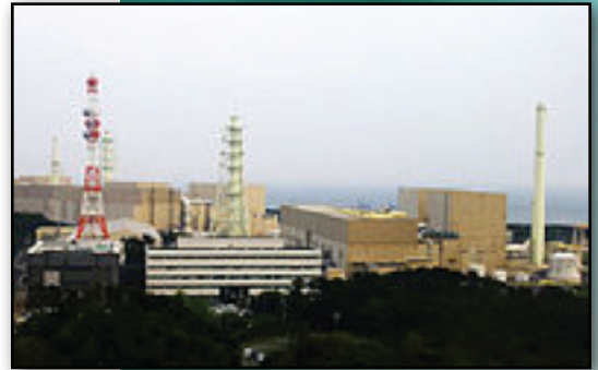
Hamaoka-5 Nuclear Power Station
