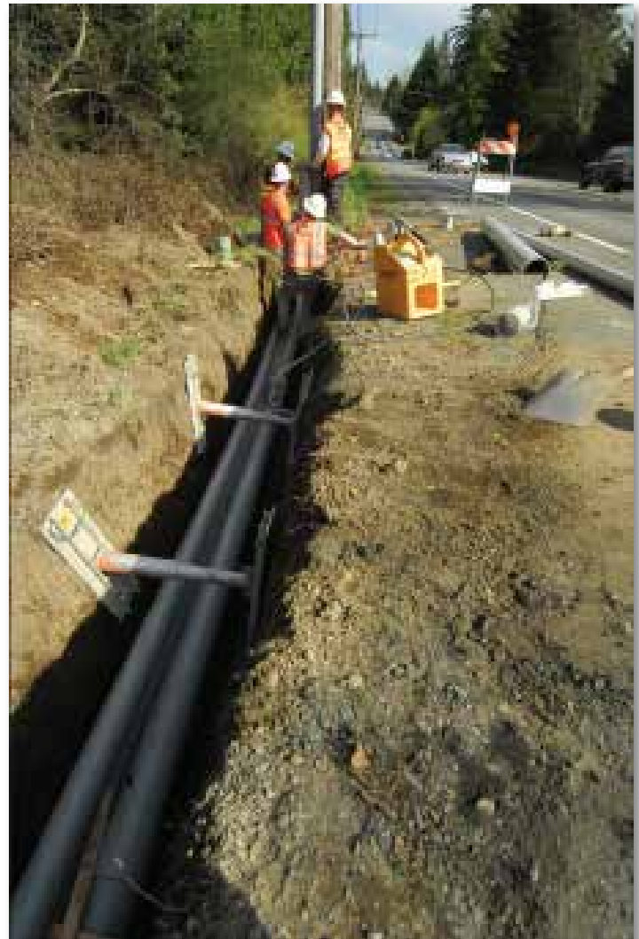
Figure 3 – An economical option for grid “hardening” may be to bury selected portions of the system.
