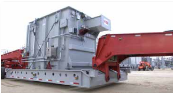
Figure 9 – Rapid deployment of “recovery transformers” could prevent sustained outages to large numbers of customers. (Photo: DHS S&T)
