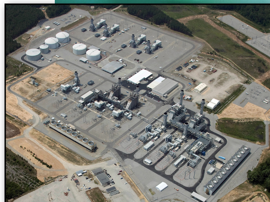
The project involved units 1–4 and 7–8 at Duke Energy's 1,904-MW Sherwood H. Smith, Jr. Energy Complex in Hamlet, NC.
