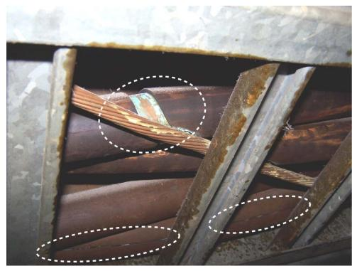
Note: Corrosion of tray and shield are likely from chlorine released by the aging of the neoprene. The jacket has turned brown from the original black and is very hard. The brown color of the jacket is a strong indication of exposure to elevated temperature.
