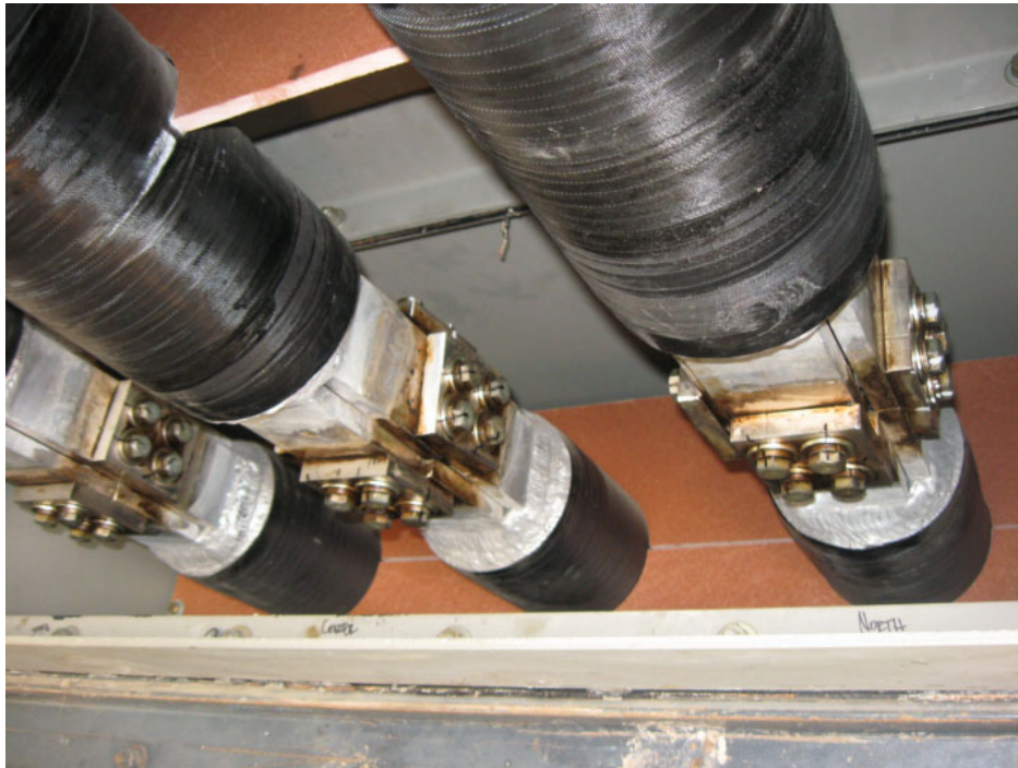
Figure 3-1 The splice plates installed at Dresden Unit 2
