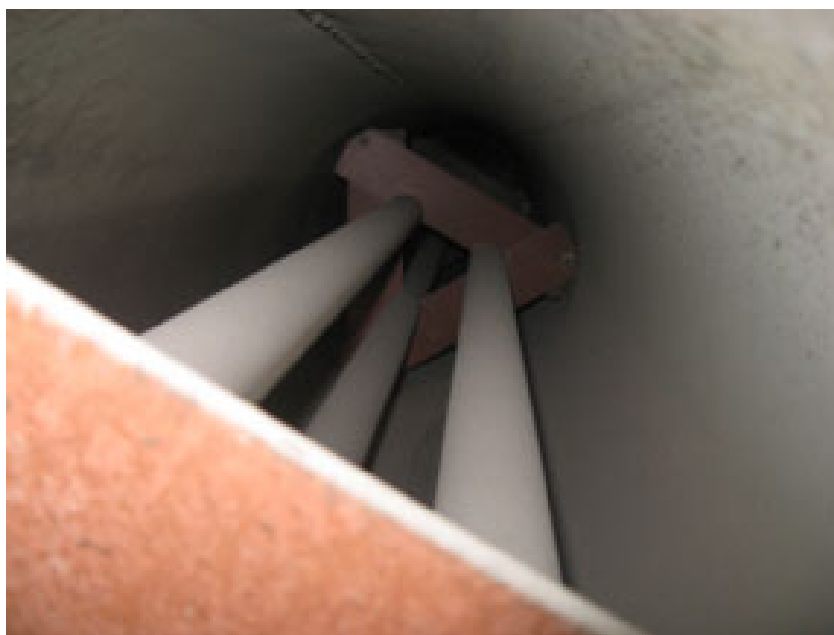
Figure 4-3 Long runs between clam shells preventing thorough cleaning
