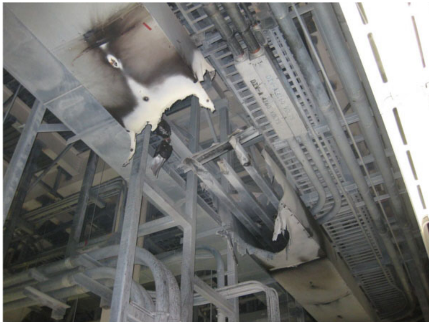
Figure 2-1 The catastrophic failure of a 6.9-kV non-segregated phase bus at a U.S. nuclear power plant
