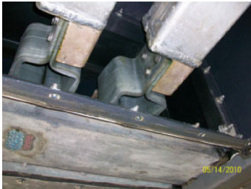
Figure 3-4 A non-segregated bus bolted flex connection, Example 2
