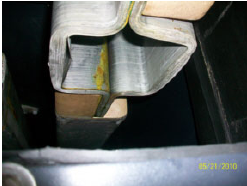
Figure 3-5 A non-segregated bus bolted flex connection, Example 3
