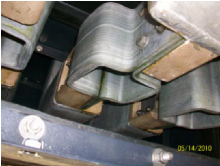
Figure 3-3 A non-segregated bus bolted flex connection, Example 1
