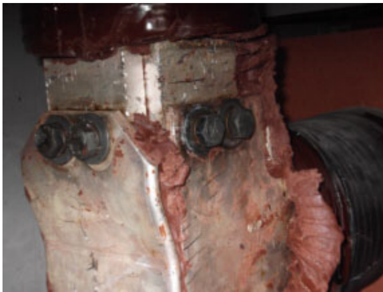
Figure 3-2 A 4-kV non-segregated bus joint at Quad Cities
