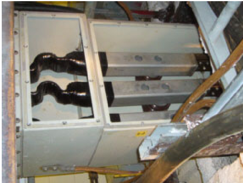
Figure 3-6 Non-segregated bus bolted connections
