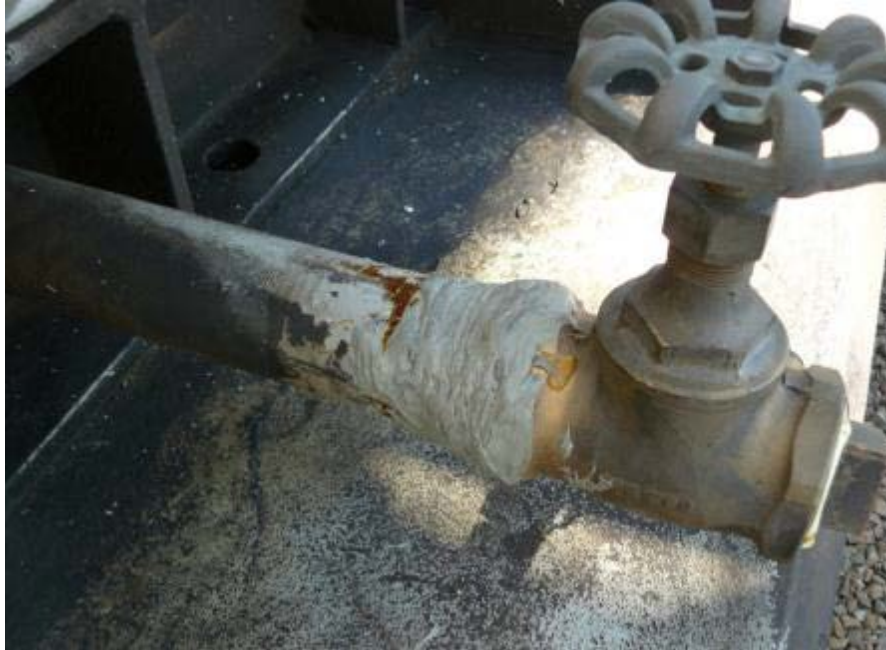
Figure 6–2 In-house repair utilizing epoxy.
