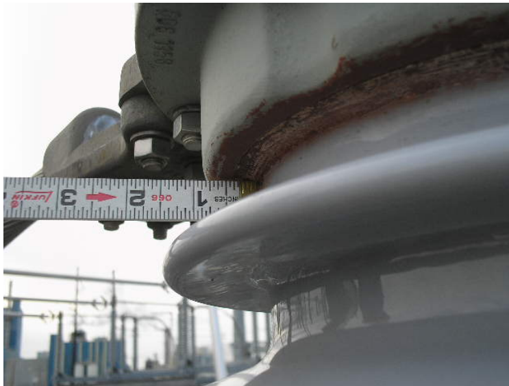
Figure 6–8 Precise measurements are taken prior to designing the clamp.
