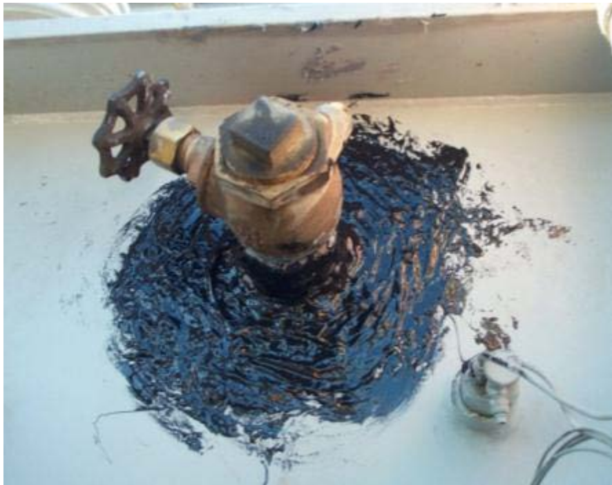
Figure 6-1 In-house repair utilizing epoxy.
