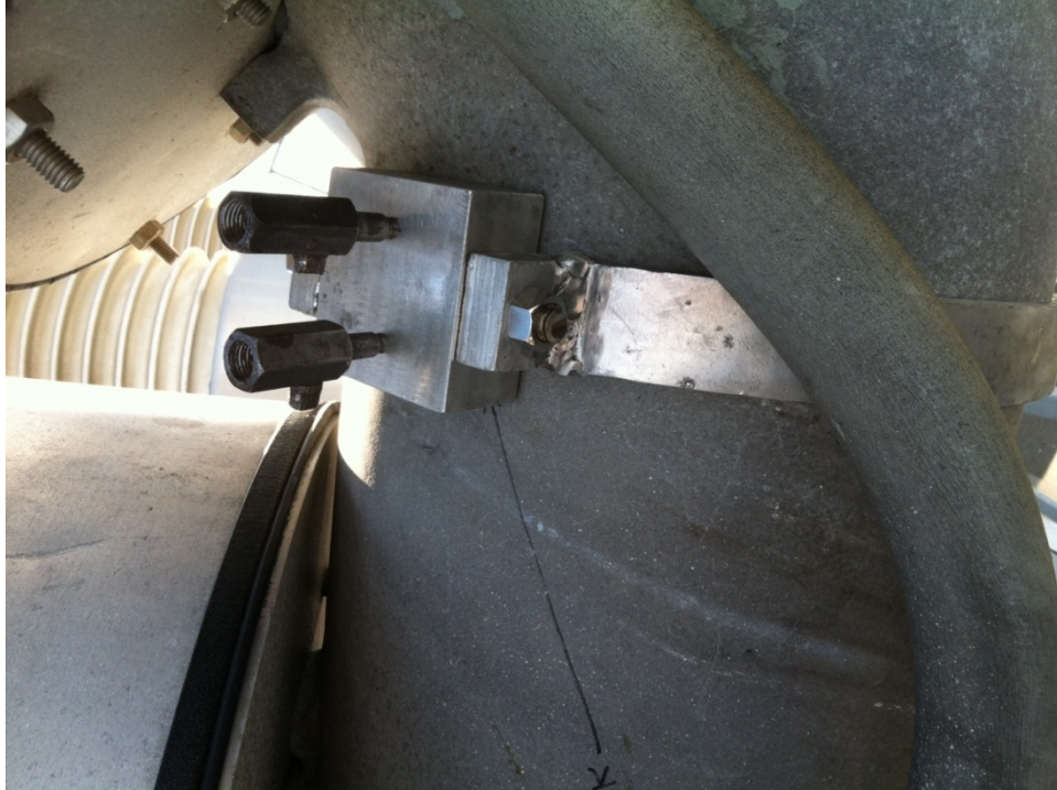
Figure 6–6 Clamp is installed over the leak with injectors to facilitate sealant injection.
