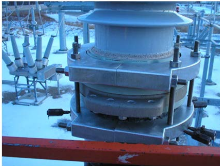
Figure 6–10 The clamp is installed over the leak.
