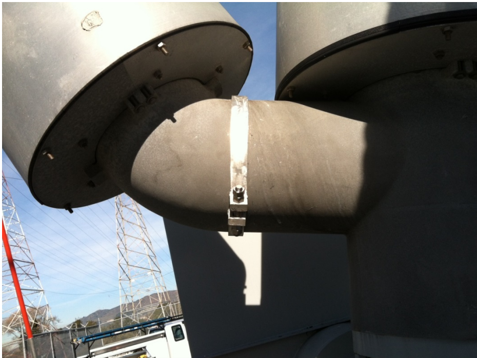
Figure 6–7 Injectors are removed and pipe plugs are installed.
