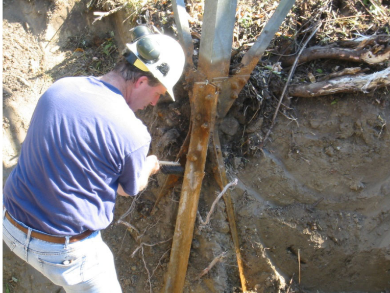
Figure 2-1 Well drained soils are typically neutral in pH and do not support localized corrosion
