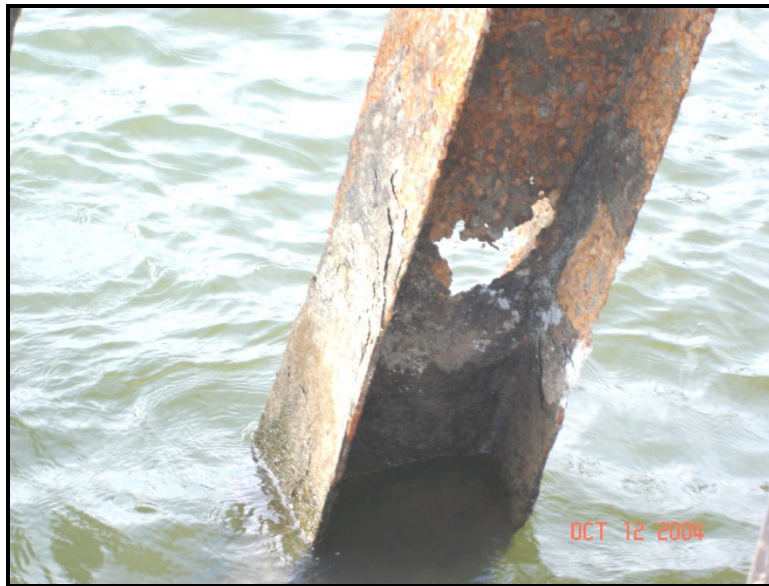
Figure 2-4 Steel H Pile installed in a marine environment
