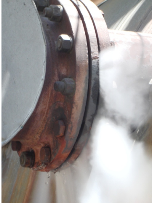
Figure 1-6 Temporary leaks of high-energy steam can degrade nearby cables
