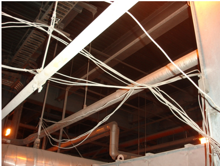
Figure 1-4 Poorly run DCS cable back-fit modification
