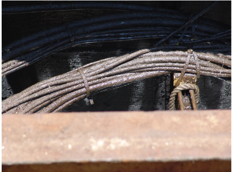
Figure 1-2 Oil-soaked cable in below-grade cable vault
