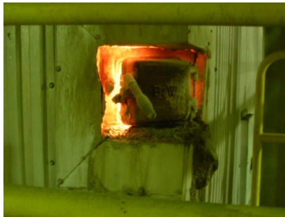
Figure 1-5 Boiler inspection port exhibits extreme radiant heat
