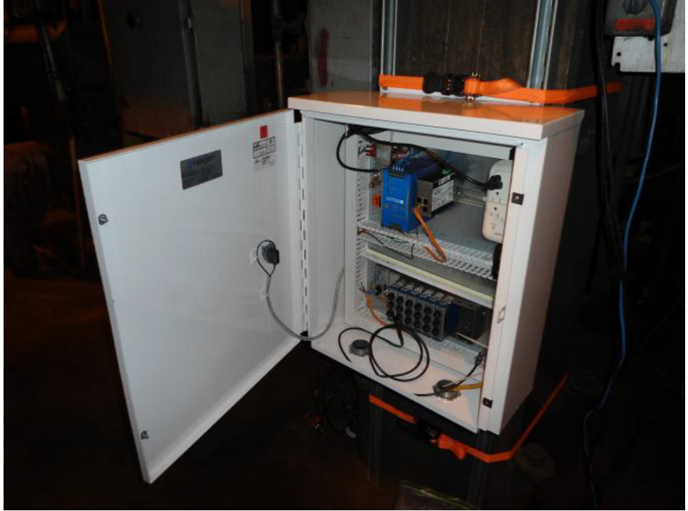
Figure 2-4 Vibration monitoring system
