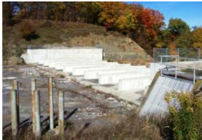
Figure 1-12 Energy dissipater [12]
