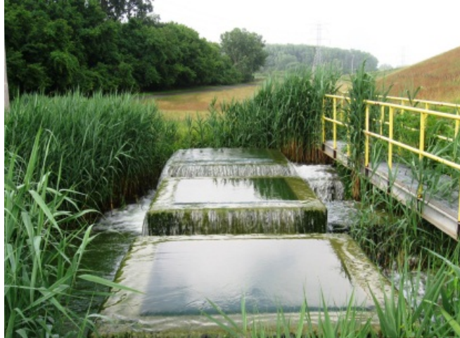
Figure 1-11 Aerator at discharge (courtesy DTE Energy)
