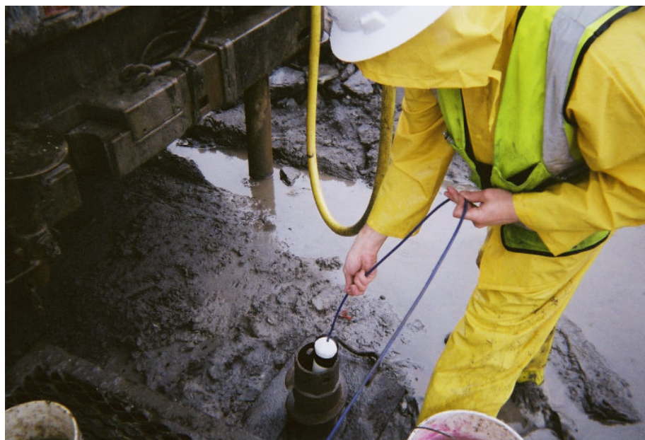
Figure 8-10 Vibrating wire piezometer being lowered down drill hole
