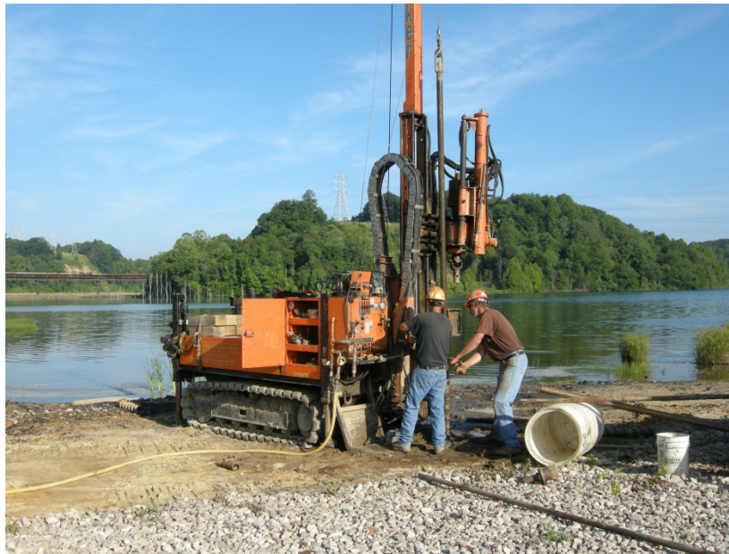
Figure 5-1 Tracked drill rig being used at a fly ash pond
