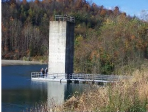
Figure 1-9 Decant structure [12]
