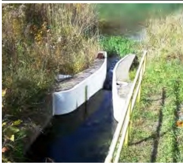
Figure 1-14 Parshall flume [12]
