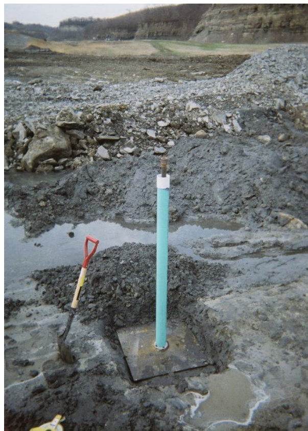
Figure 8-9 Settlement plate with PVC riser sleeve
