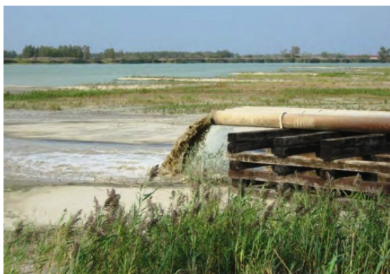
Figure 1-2 Fly ash sluice lines [11]
