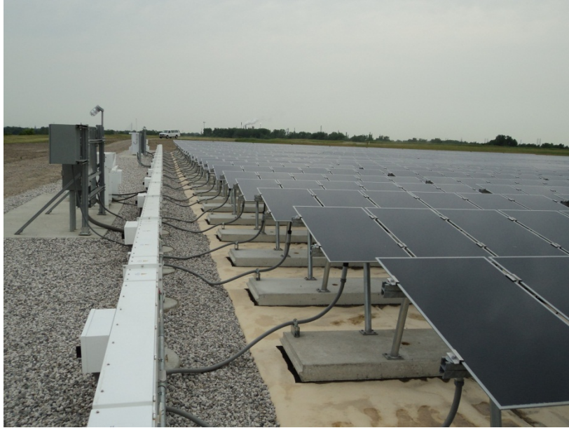
Tracking rigid panel system installed on a lined brownfield site. Photo provided by American Environmental Group [9]
