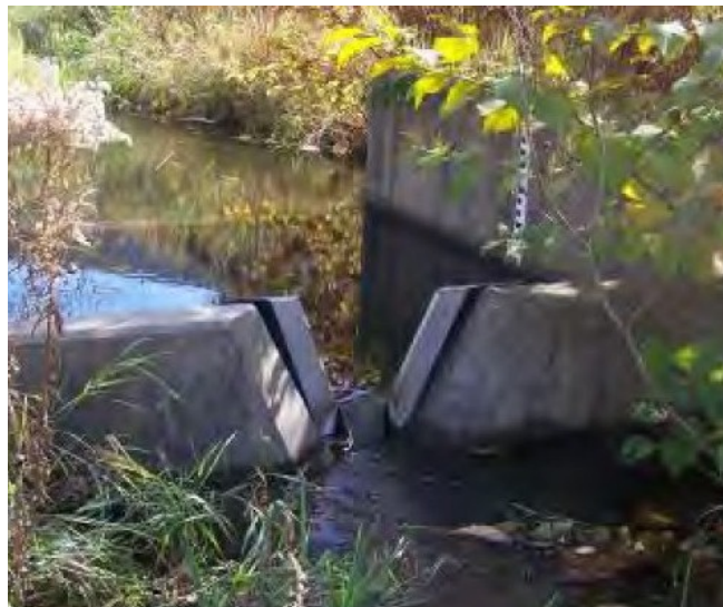
Figure 1-15 V-notch weir [12]
