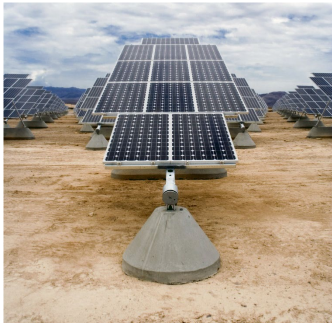
Photo of a ballast foundation system from Nellis Air Force Base, Nevada (courtesy of SunPower Corporation)
