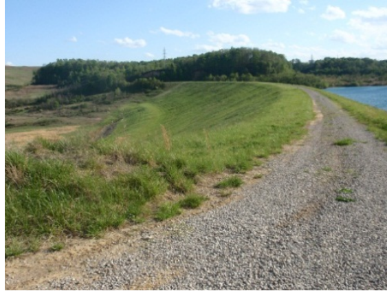
Figure 1-7 Containment structure (courtesy of AEP)
