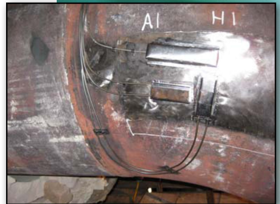
Installation of high-temperature strain gauges on P91 at TECO's Bayside Plant
