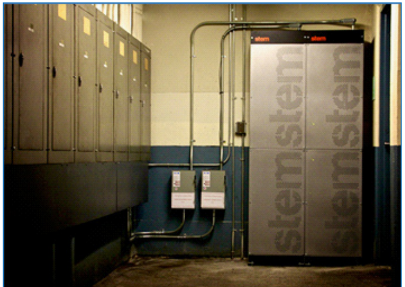
36-kW Stem PowerStore Installation (Source: Stem)
