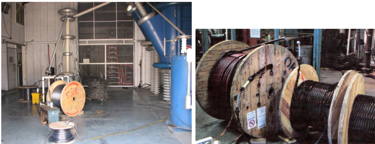
Figure 2-2 High-voltage test setup
