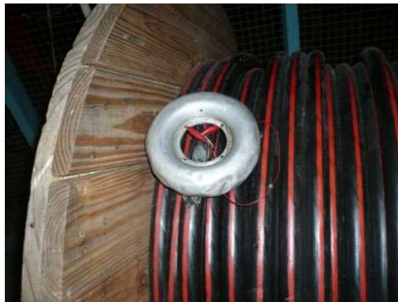
Figure 3-2 Hole in the cable insulation covered with a donut—compare to Figure 2-4
