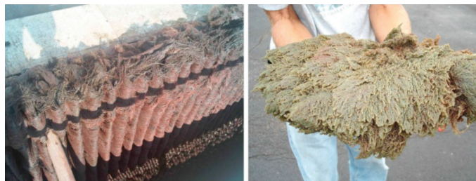
Fouling of a trash rack (left) at Ft. Myers Plant (photo courtesy of Florida Power & Light) and (right) a large sample of bryozoans taken from the forebay of a nuclear power plant (photo courtesy of Bryo Technologies).
