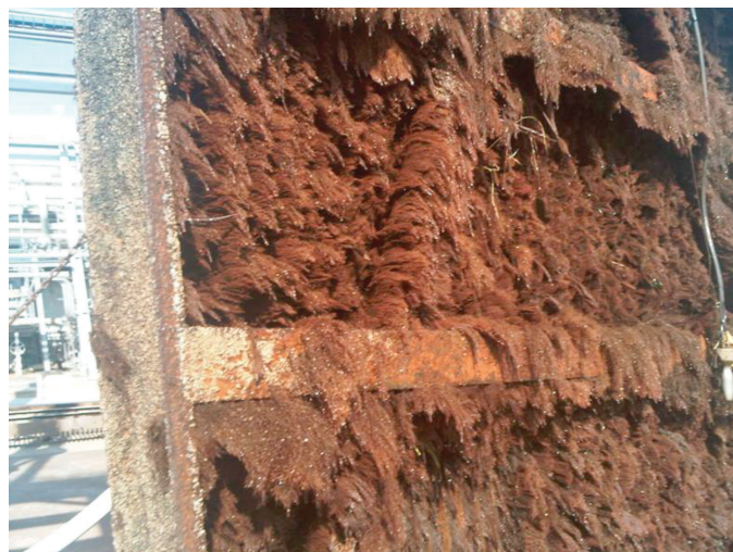
Figure 3. Fouling of a trash rack at Florida Power and Light Ft. Myers Plant (Image courtesy FP&L).
