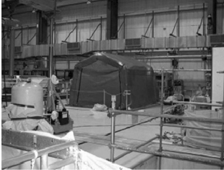
Figure 3-4 Tent completely enclosing an FME zone
