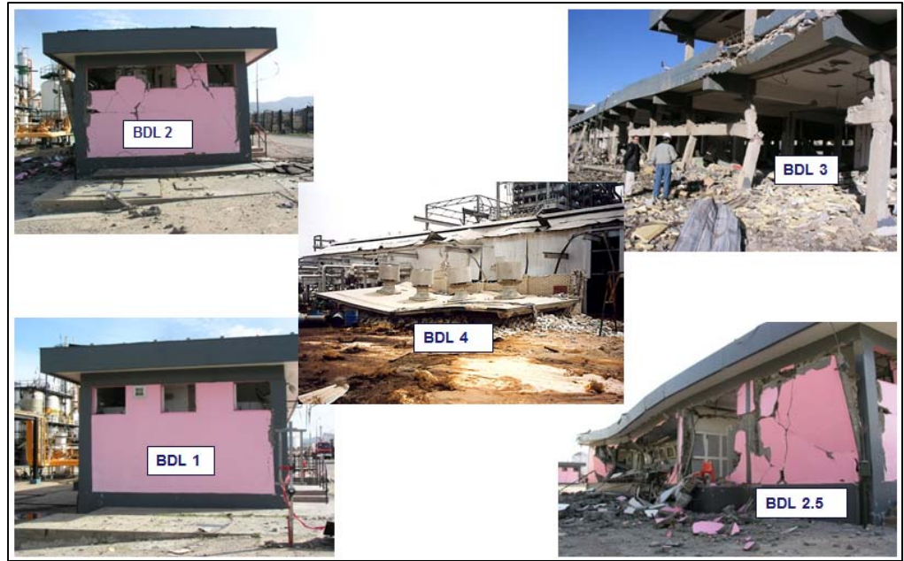
Figure B-4 Building Damage Levels (BDL)
