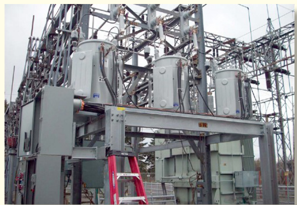
Figure 3 – National Grid has Installed the DX3 Pulsar PLC System at a Substation in Upstate New York (Photo Courtesy of National Grid)
