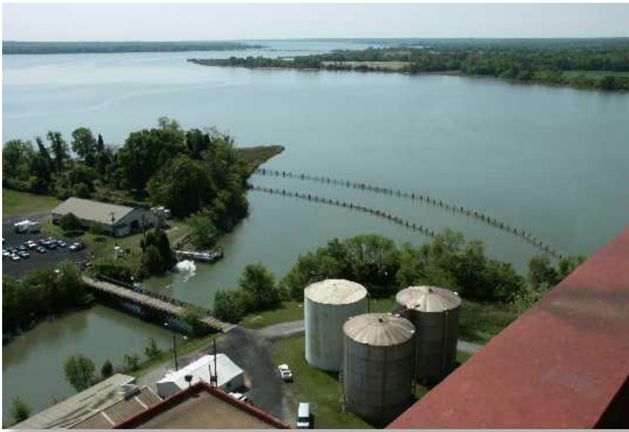
Figure 4 – Barrier net (double net system with exterior mesh of 1.5 in and interior of 0.75 in stretch mesh) at the mouth of the Chalk Point Generating Station CWIS (Image courtesy D. Bailey)
