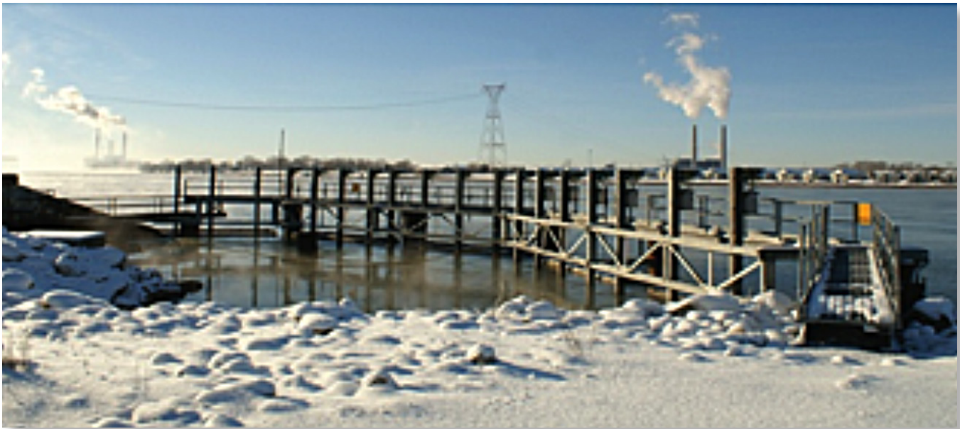
Figure 3 – Sound and strobe light barrier used at Ontario Power Generation's Lambton Station (Image from Someah 2011).
