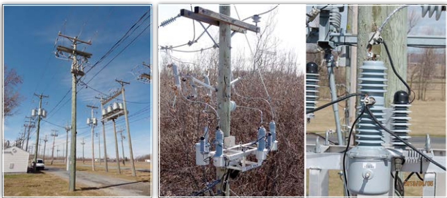
Left is sectionalizing switch; middle and right show autoground switch
